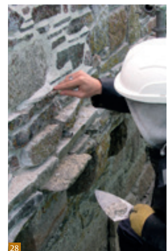
Fig. 28 Repointing rubble masonry.
