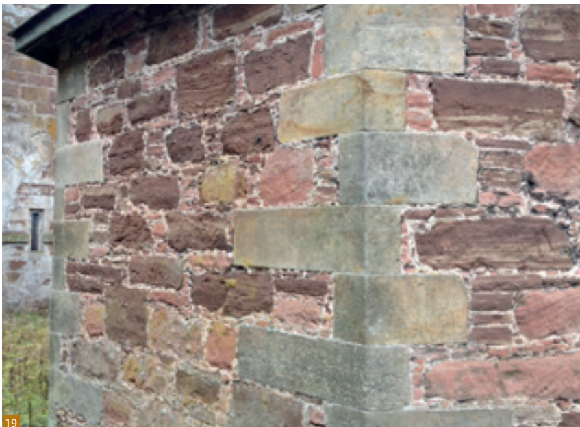
Fig. 19 The use of lime mortar with multiple stone types.
