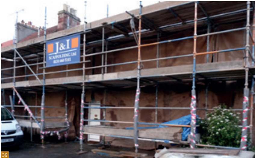
Fig. 39 Full façade protection of lime render with hessian covers (© G. Frew).
