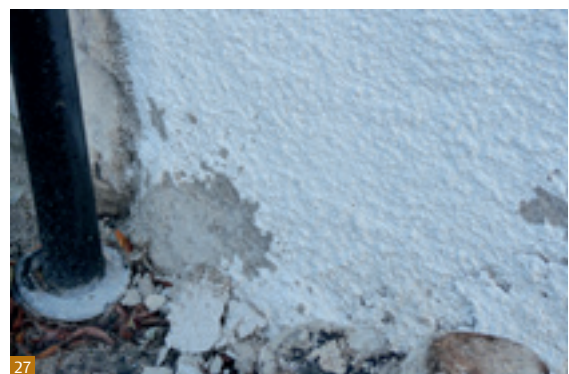
Fig. 27 Frost damage to lime harling.
